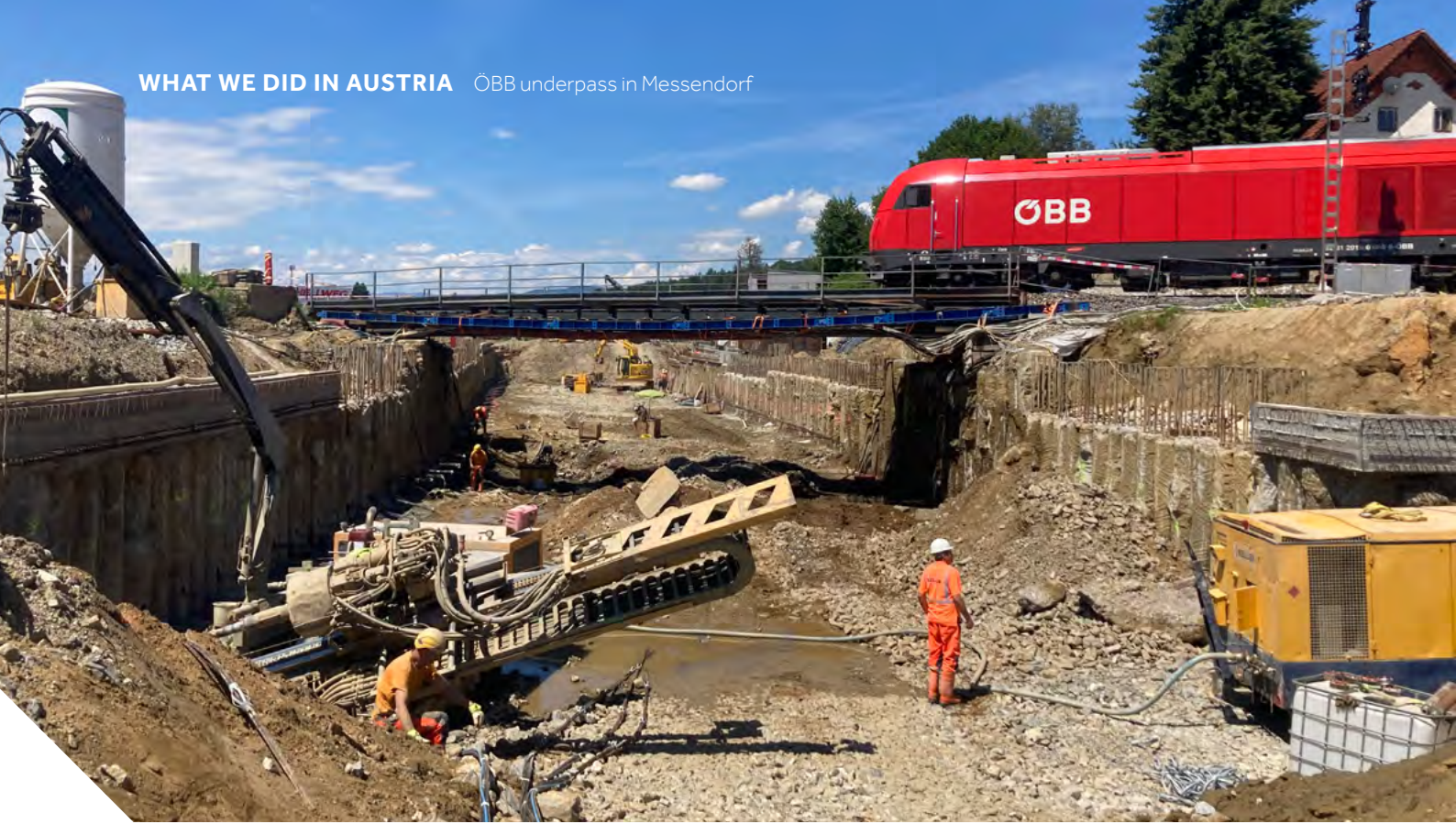
CONSTRUCTION OF THE TEMPORARY ANCHORS
