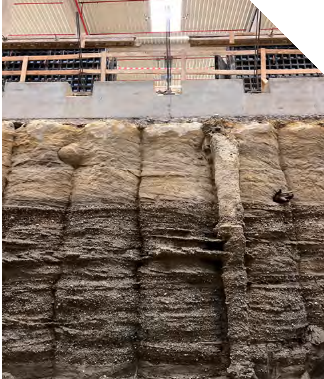
THE EXPOSED SOILCRETE WALL
