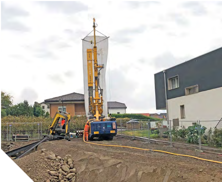
VERTICAL DRILLING – KING POST SOLDIER WALL
