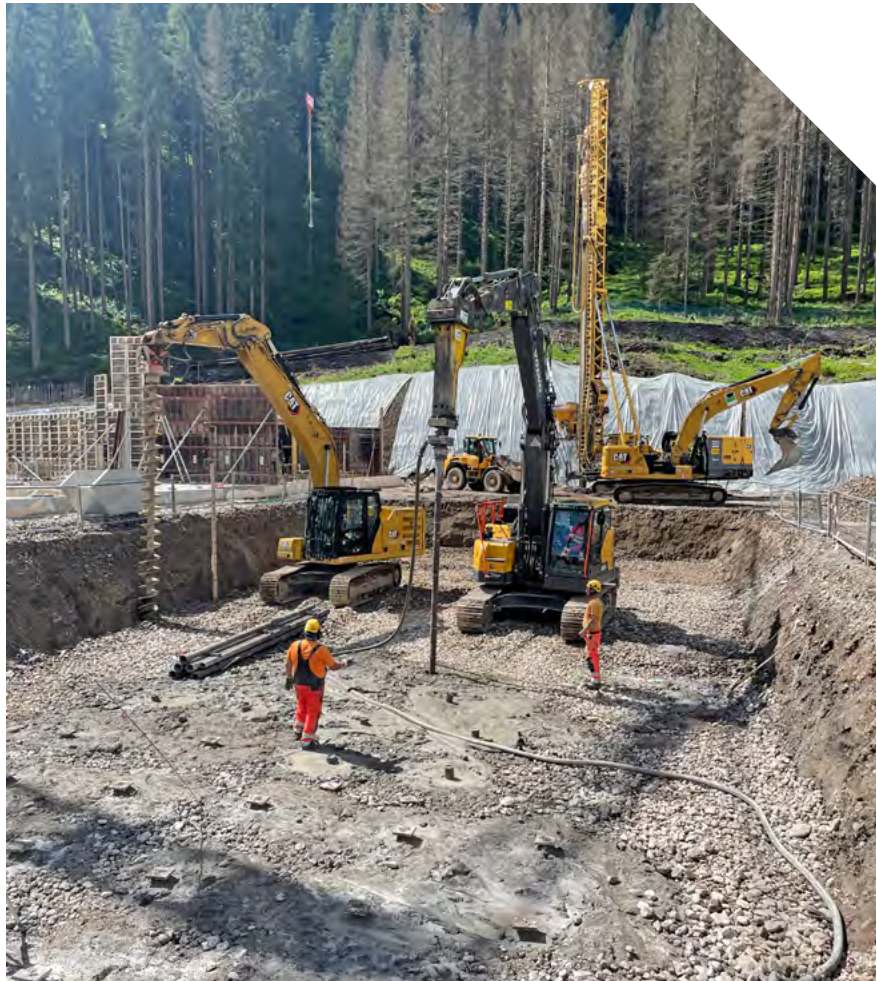
INSTALLATION OF DRIVEN PILES
